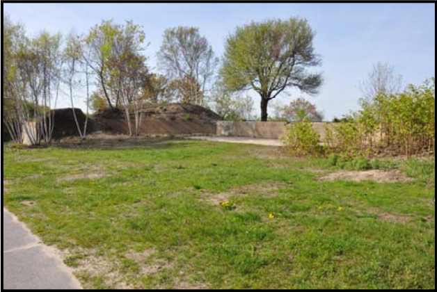
3.1 The Cliffside Site at Battery Hobart.
