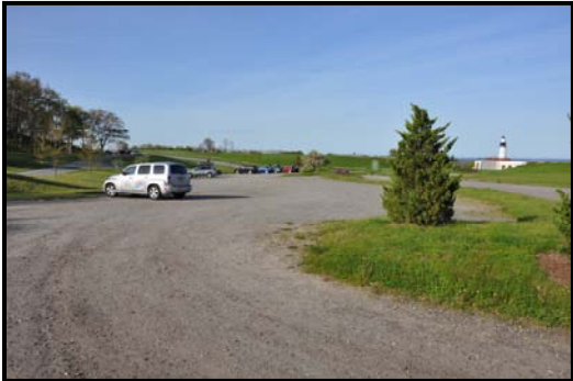
9.3 Central parking lot.
